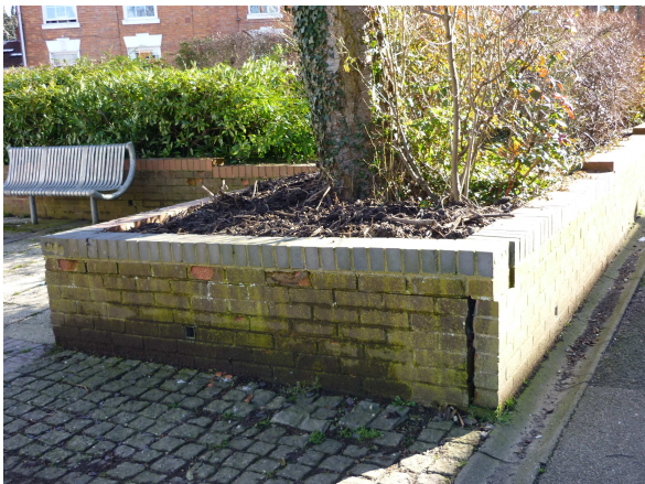
We have secured funding to work with Oxfordshire Highways and Banbury Town Council to undertake streetscape improvements in Centre Street and East Street, Grimsbury
