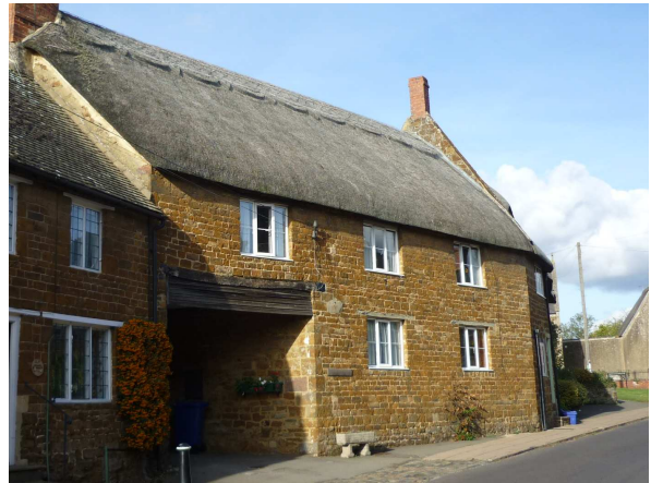
Former Royal Oak public house in Adderbury, now a dwelling with rear garden and off-street parking
