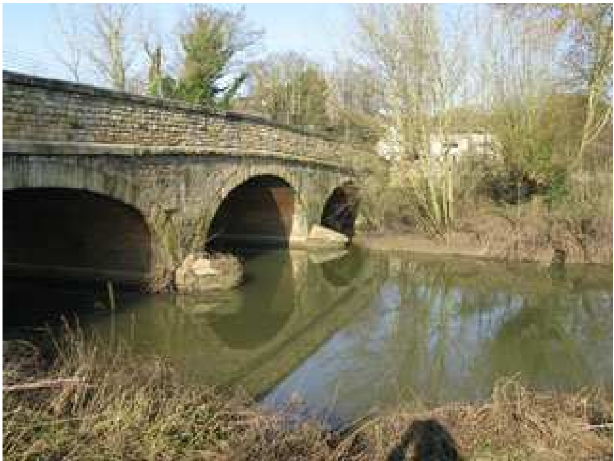
The historic bridge over the River Ray, Islip
