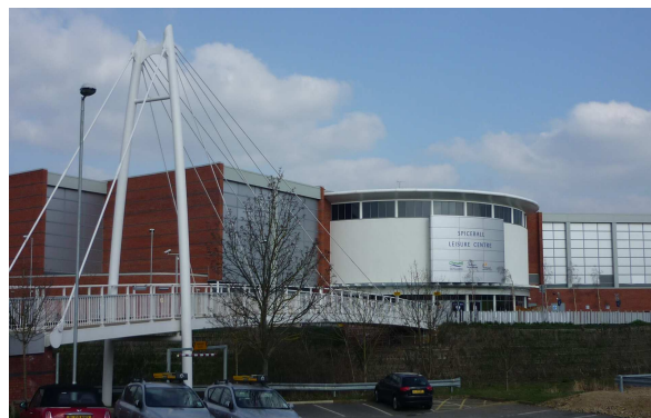
Above: The new Spiceball Sports and Leisure Centre linked to the town centre by bridge in accordance with our Design Brief
