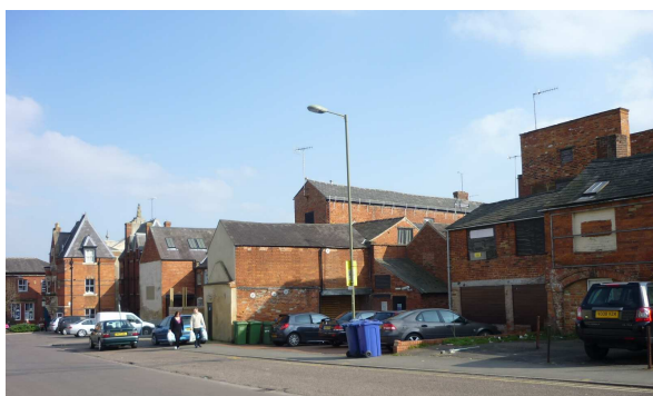
Bolton Road, Banbury, where a retail-led regeneration scheme is being promoted by the Council which will integrate with Parsons Street and Corn Hill
