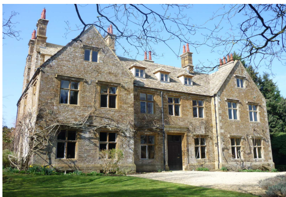
The Grange Adderbury, recently restored
