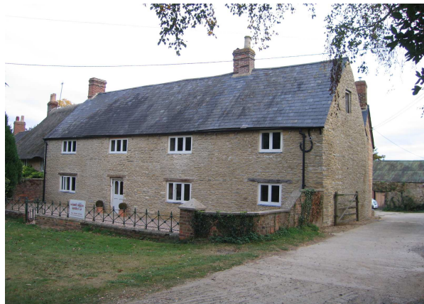
Above: Montague Farm, Hethe (grade II), after restoration
