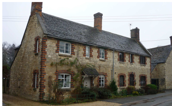
Springdale & Bishop's Cottage, non-designated heritage assets in Kirtlington; former Estate cottages where the window and door openings are framed in local red brick, with the burnt headers creating an attractive chequer board effect, that is highly locally distinctive
